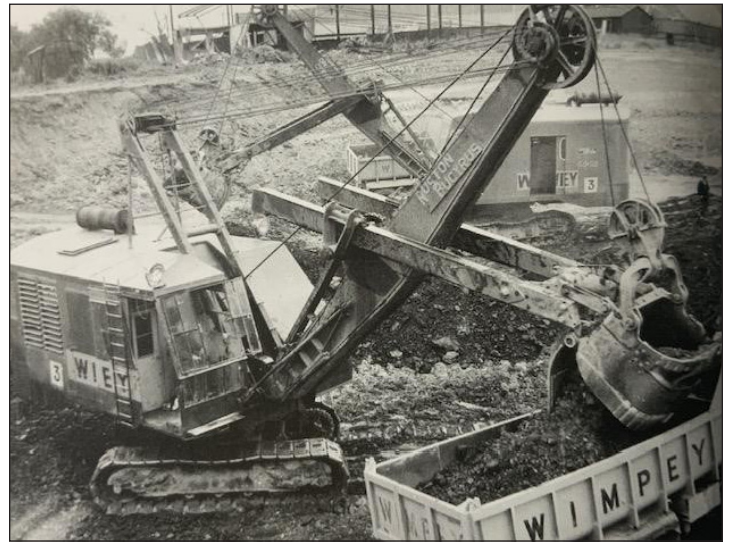
A Ruston Bucyrus 54RB at work in the U.K. Note the sign on the boom.
