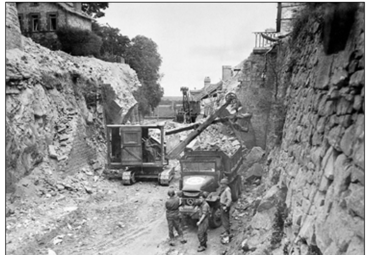
15-B Shovel with a Wood Machinery House in France
