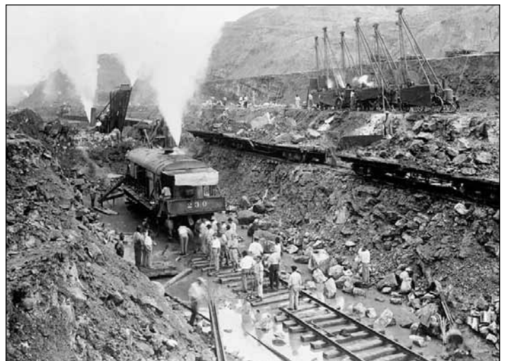
Shovels #230 and #222 “meet in the middle” of the Culebra cut on 5/20/13
