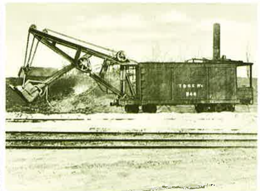
This early Bucyrus railroad shovel, carrying a 1¼ cubic yard dipper, was built in 1882.
