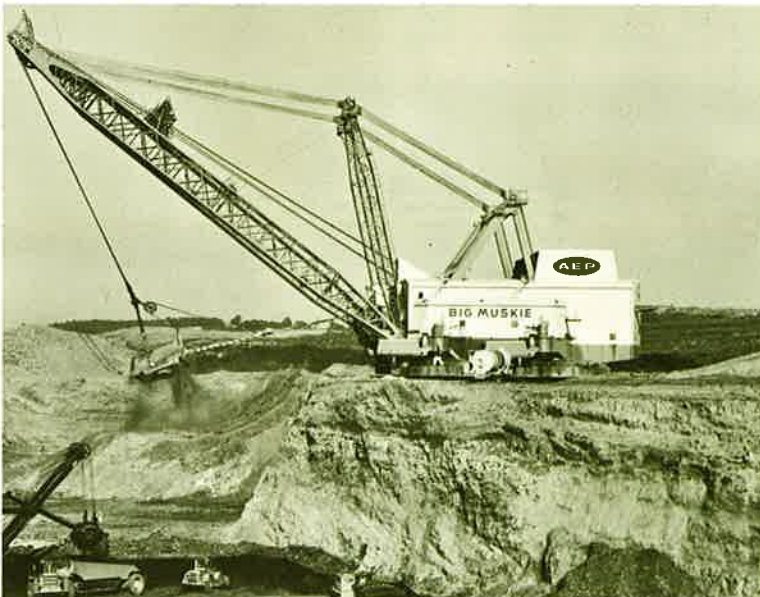
This giant $20 million walking dragline, built by Bucyrus-Erie, is the largest in the world, with a bucket capacity of 220 cubic yards.
