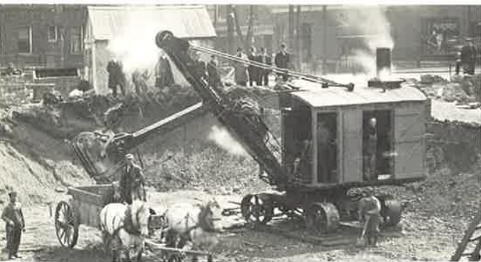
This fully-revolving Erie-B steam shovel was developed in 1914 by the Ball Engine Company, predecessor to the Erie Steam Shovel Company.
